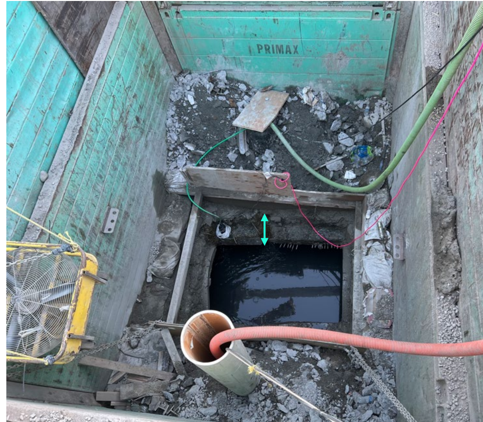
Cut Int. Ready for CIPP
