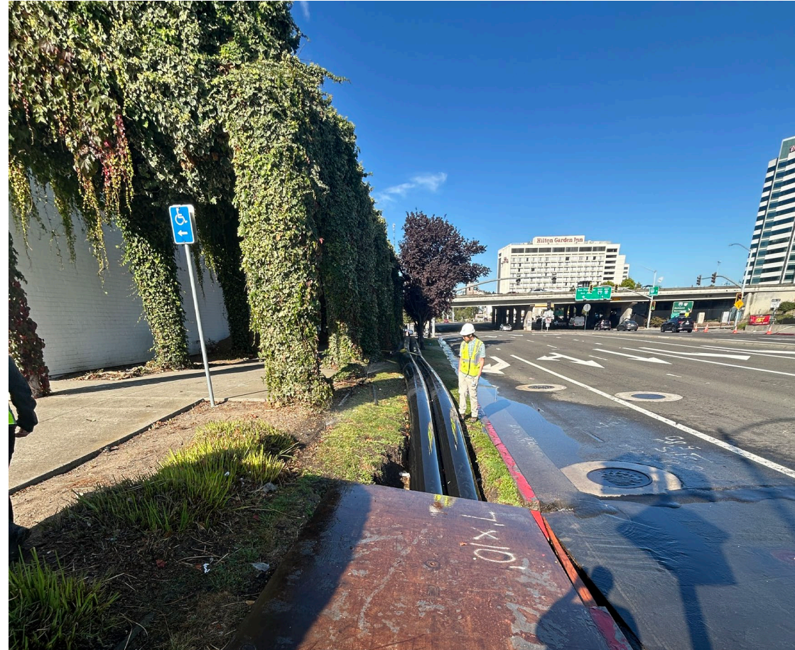
Powell Street Irrigation Leaks
