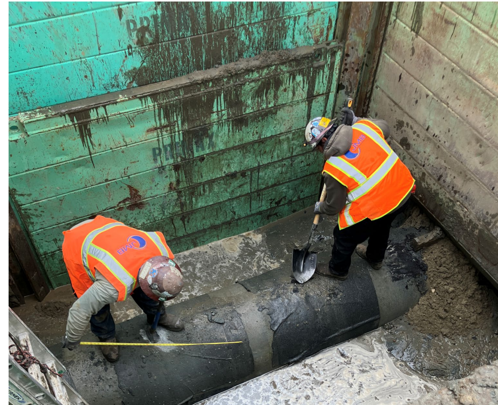
30" Storm Drain at Insertion Pit
