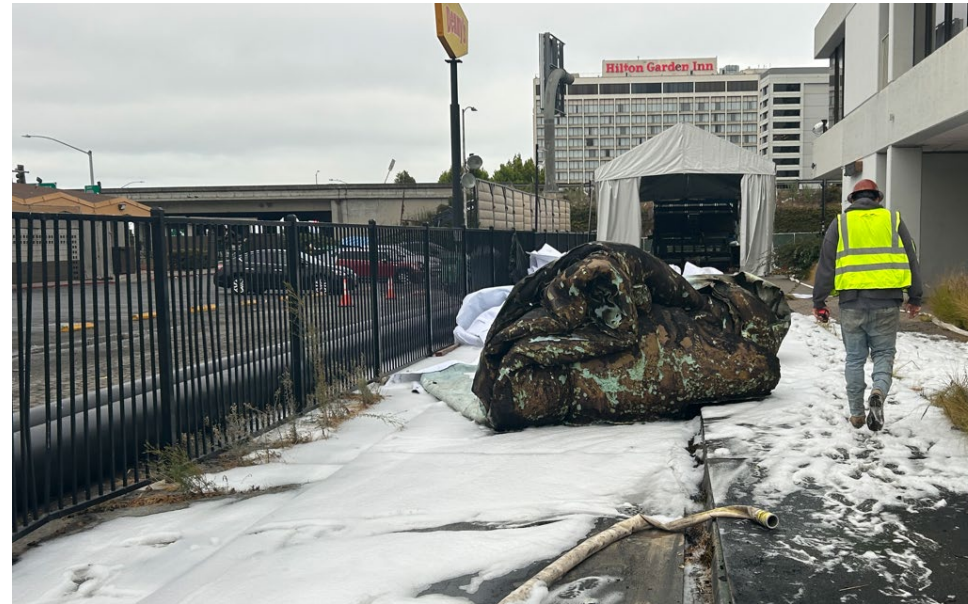
Liner at Main Staging Area
