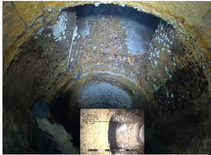
N32, from upstream view
