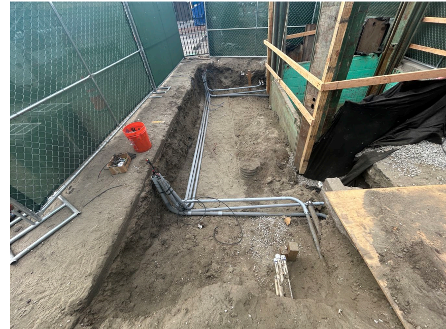
Coordinated Utility Relocations
