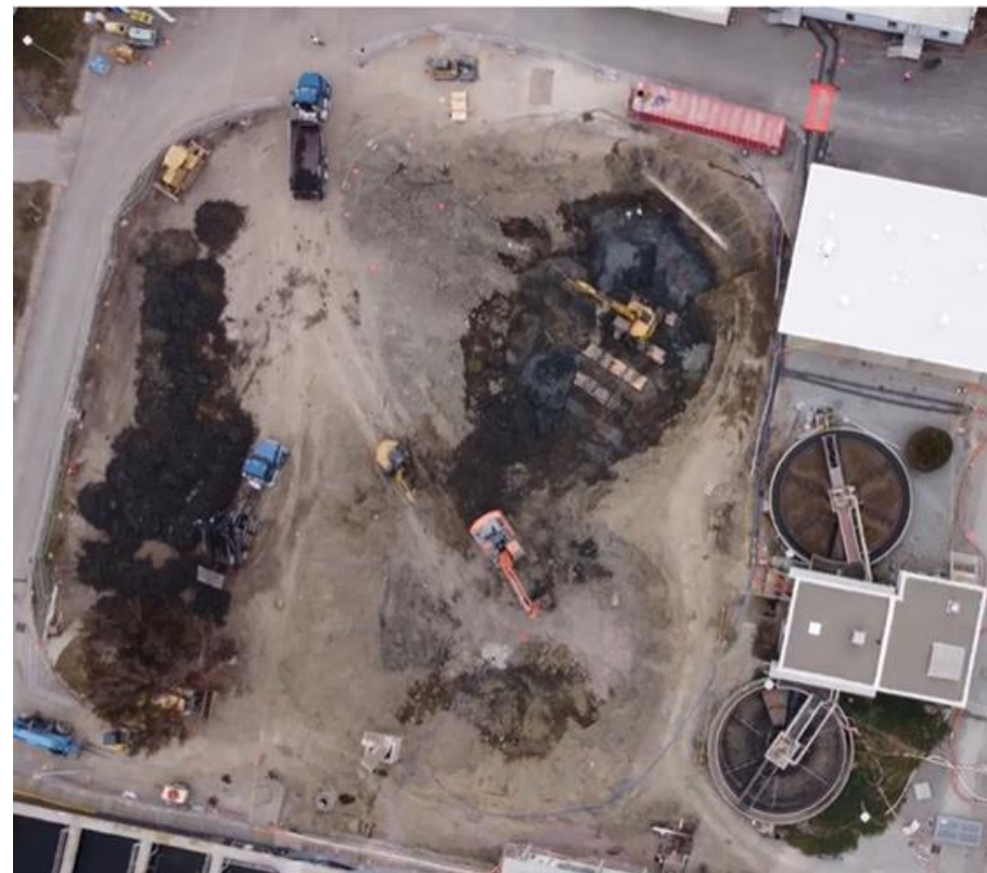
Aerial photo of Digester excavation area.
