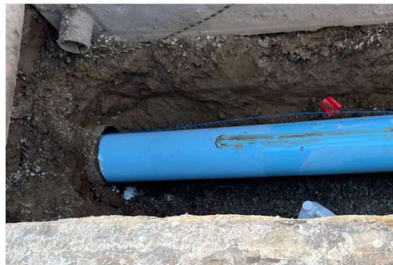
Figure 6 Typical Sliplining Access Pit for Prefused Lengths of Polyethylene Liner
