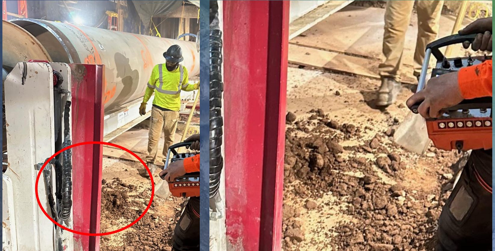
A worker shovels fragmented rock from the launch pit removed along the bore path by HHB operations.
