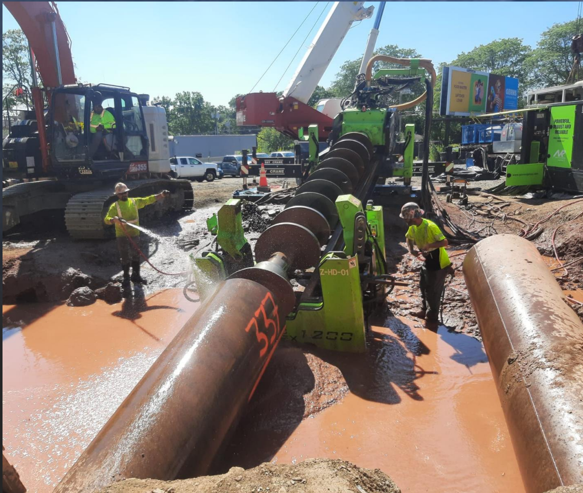
Removal of Auger String from Casing
