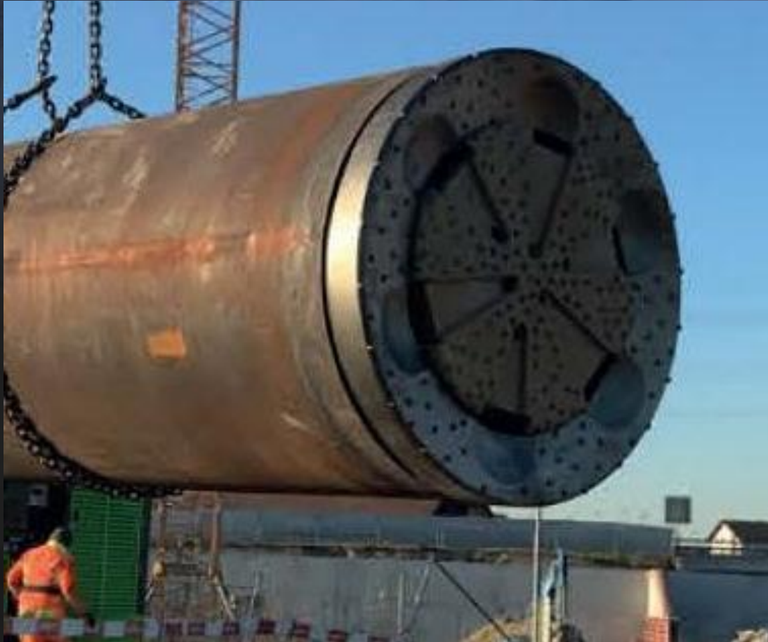
Complete cutting head of pilot bit and ring bit locked together, ready for installation.
