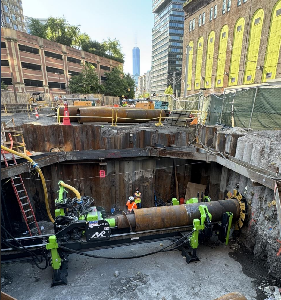
Launch Pit , the first section of casing is installed 10'
