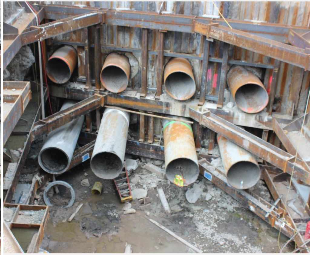
Receiving pit, looking North 8 casings installed within tolerance
