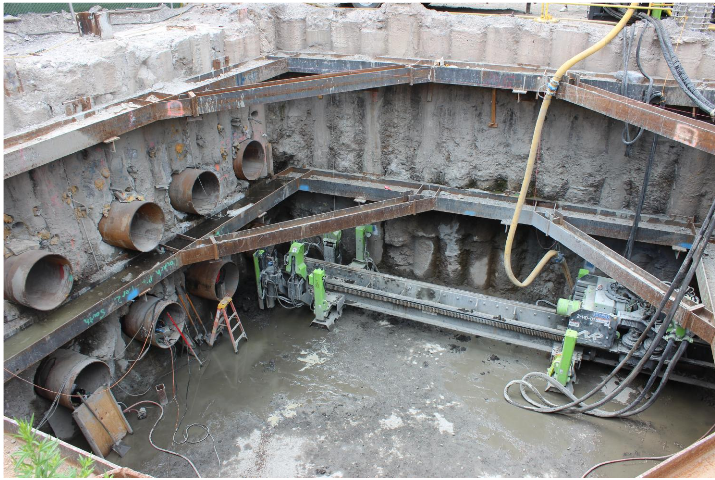
Launch Pit, looking West 8 casings installed
