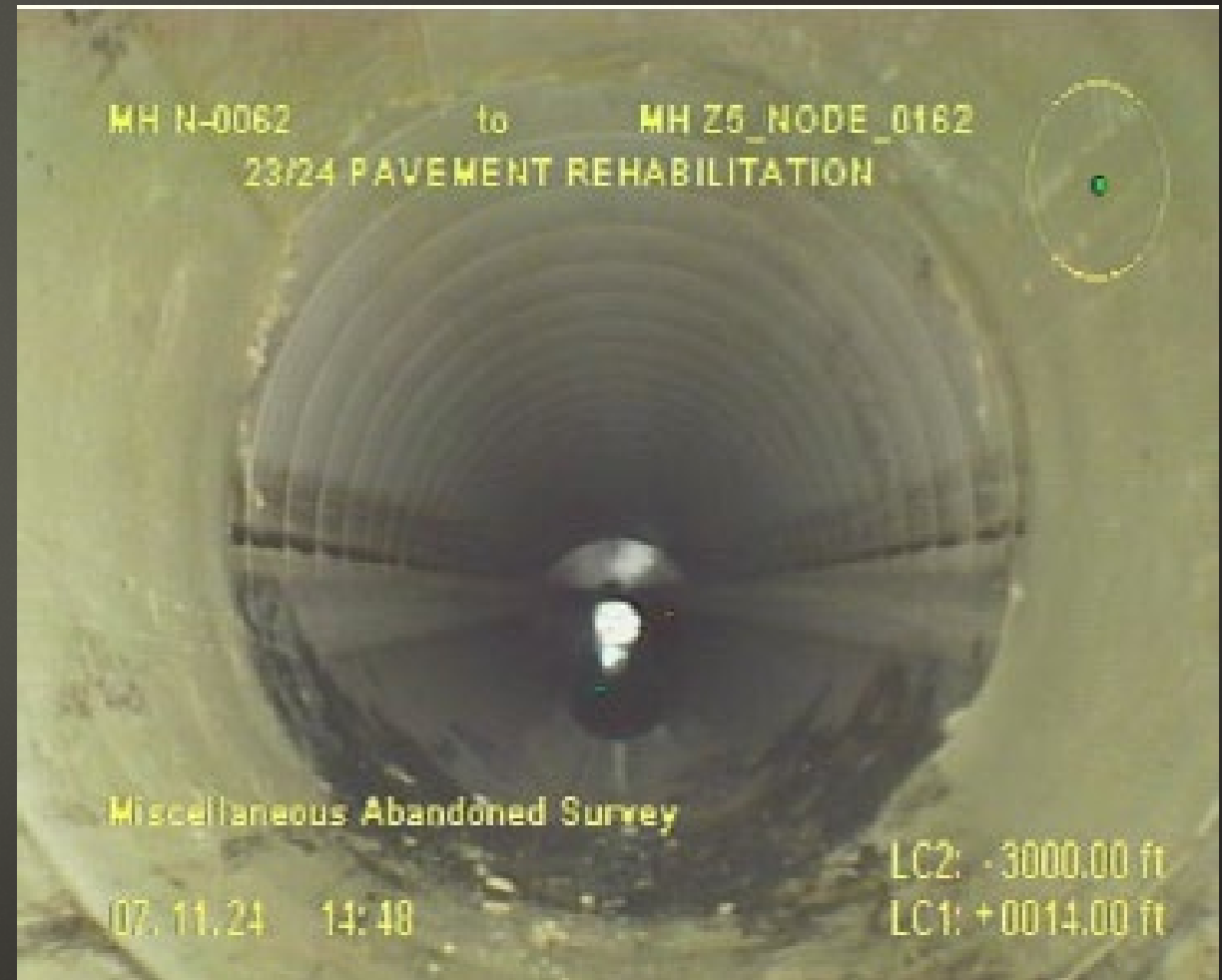
After CIPP Spot Repair
