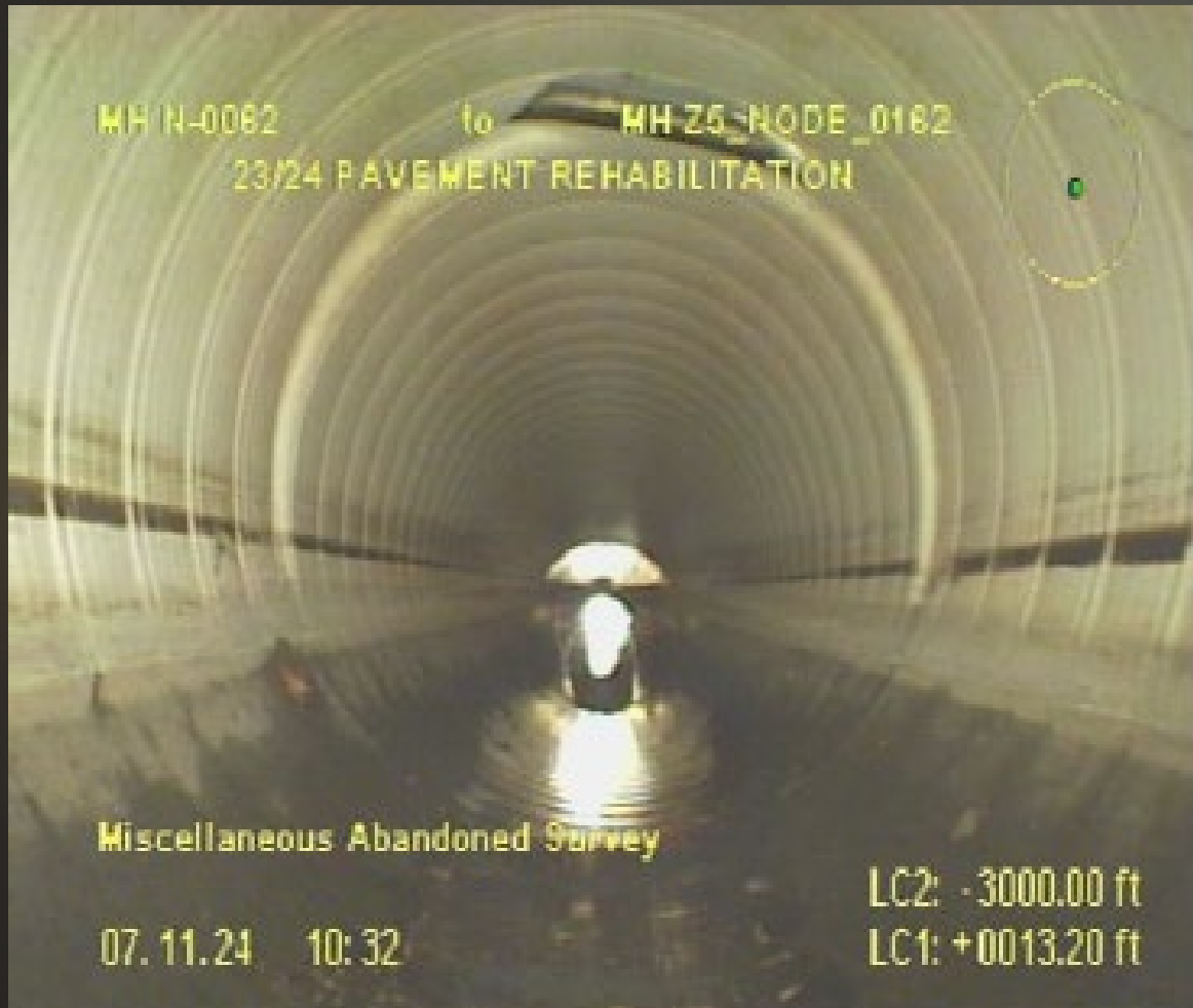
Before CIPP Spot Repair
