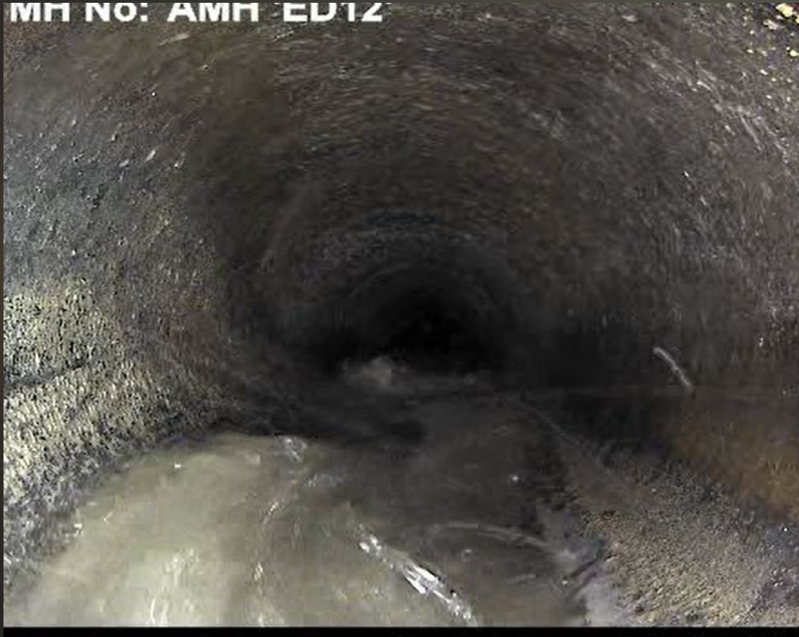
Before CIPP Lining
