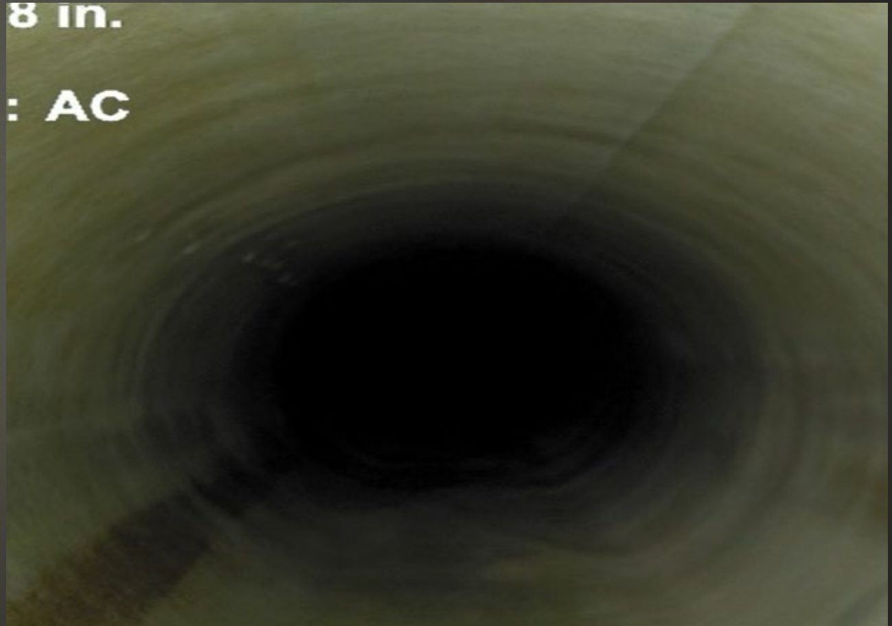
After CIPP Lining
