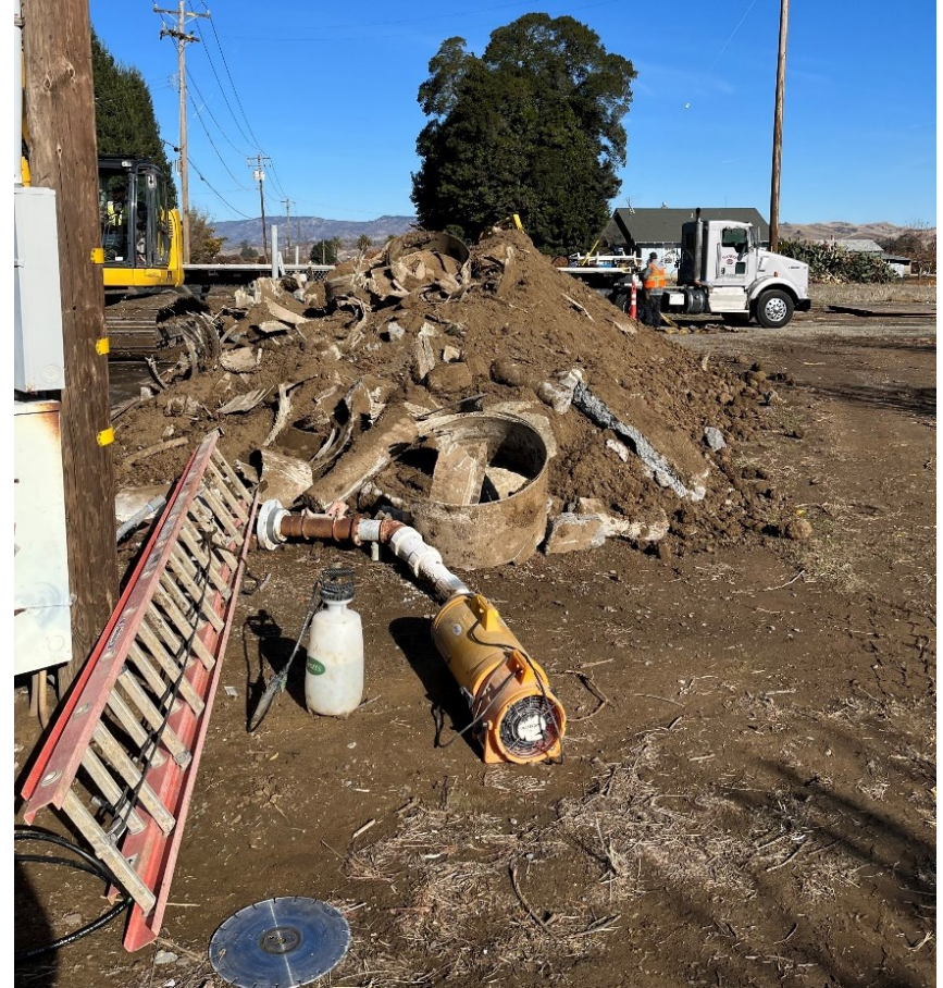
Techite removal is messy
