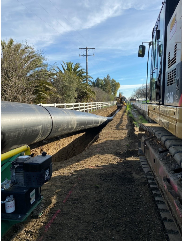
500 feet of 48" pipe in 18' corridor
