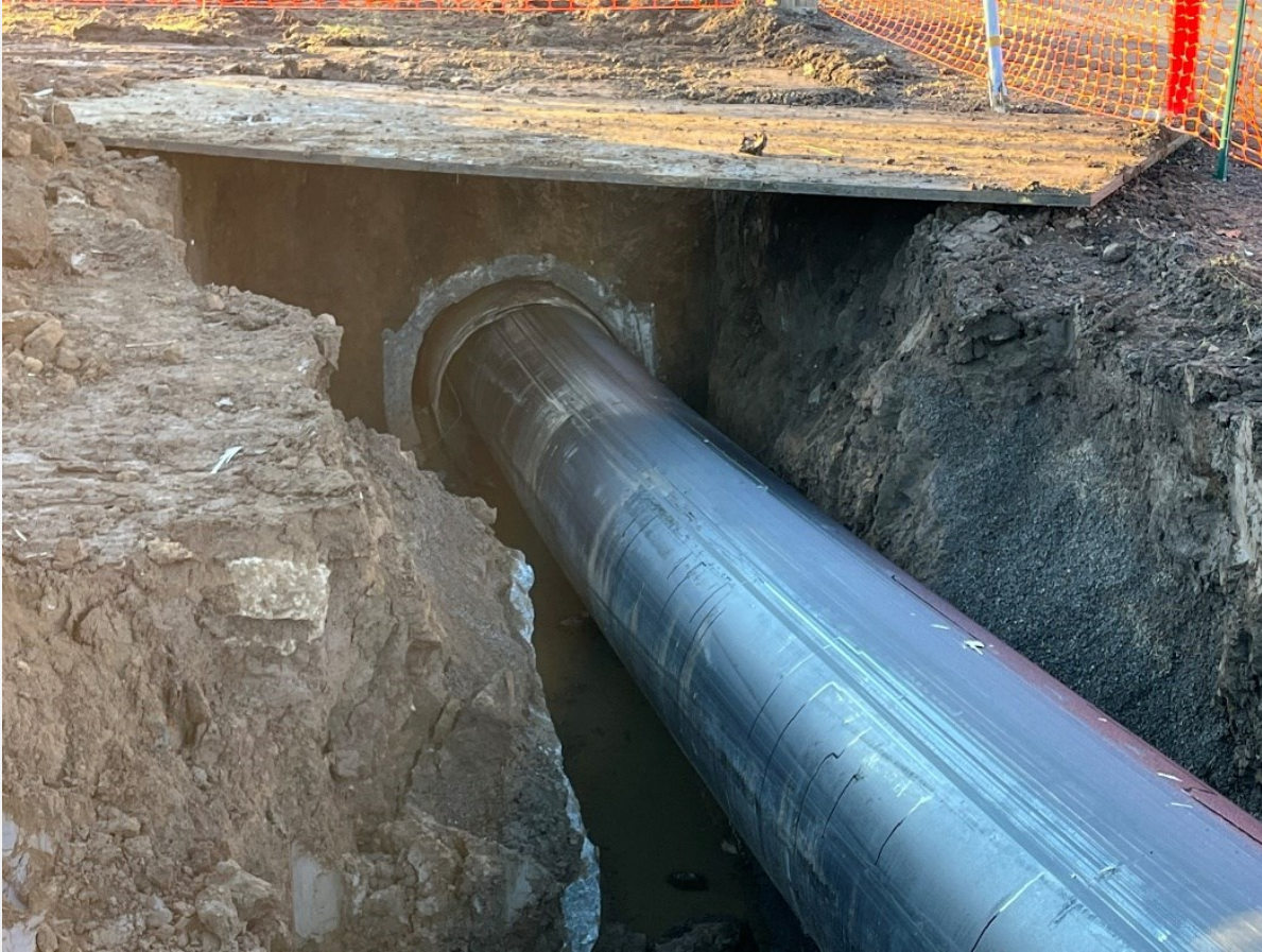
Slip-lined through Techite where possible
