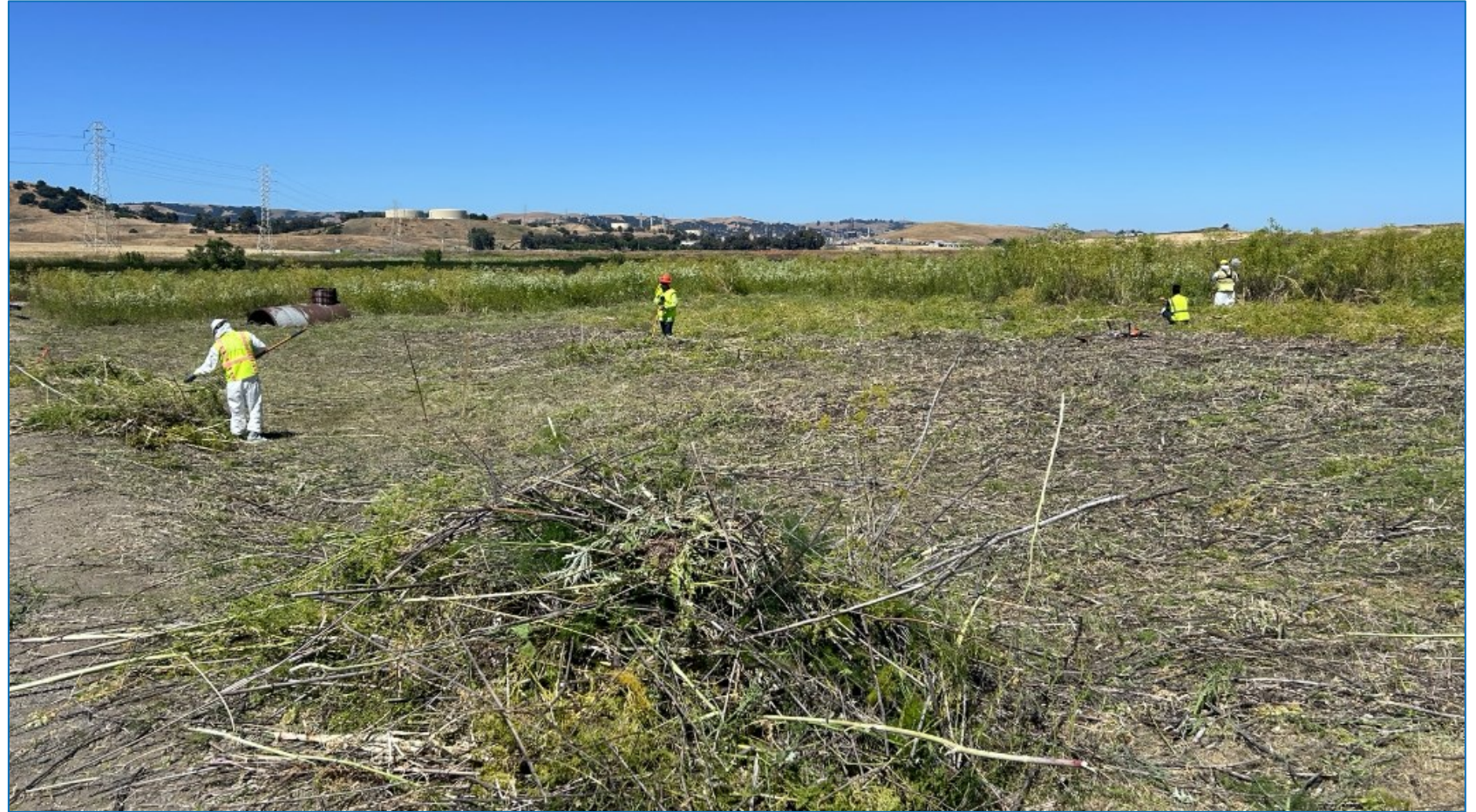
Clearing and grubbing with hand tools only!
