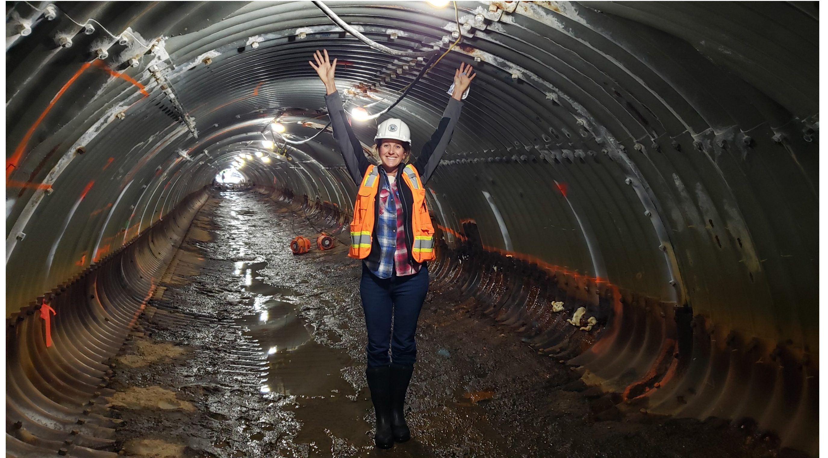
SCHOENBAR CULVERT, SHOENBAR CREEK, KETCHIKAN, ALASKA, JUNE 2024
