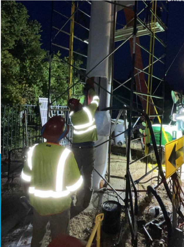
SAN TOMAS EXPRESSWAY
