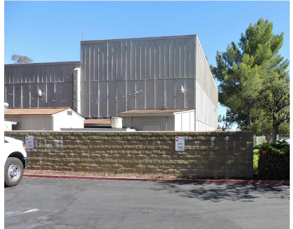
Facing North at South End of Fire Station
