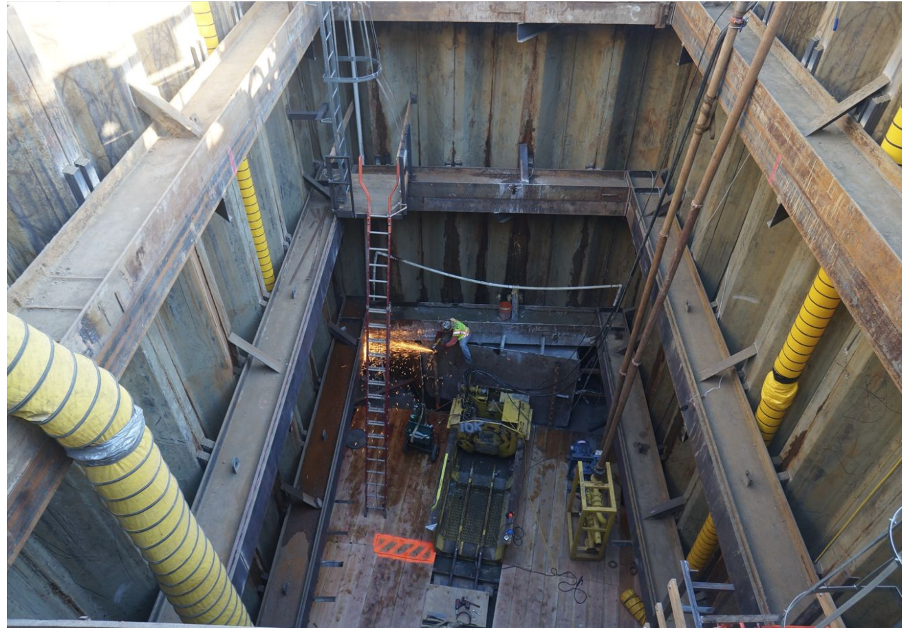
Microtunnel jacking pit
