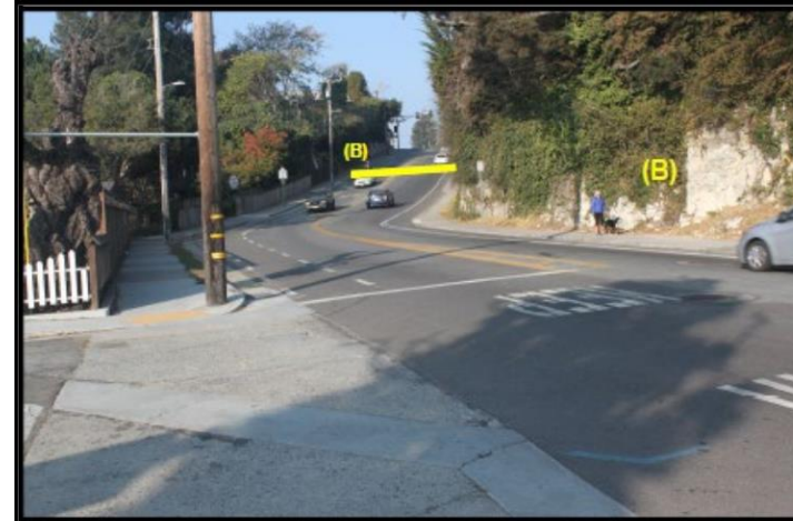
Photo 5 - Westward view along Laurel Street of the potential trenchless installation "3" of the culverted Bay Creek (A; approximated in yellow). Light-colored and relatively sedimentary soft bedrock (Purisima Formation; B) is exposed in roadcuts upslope and downslope of the crossing.
