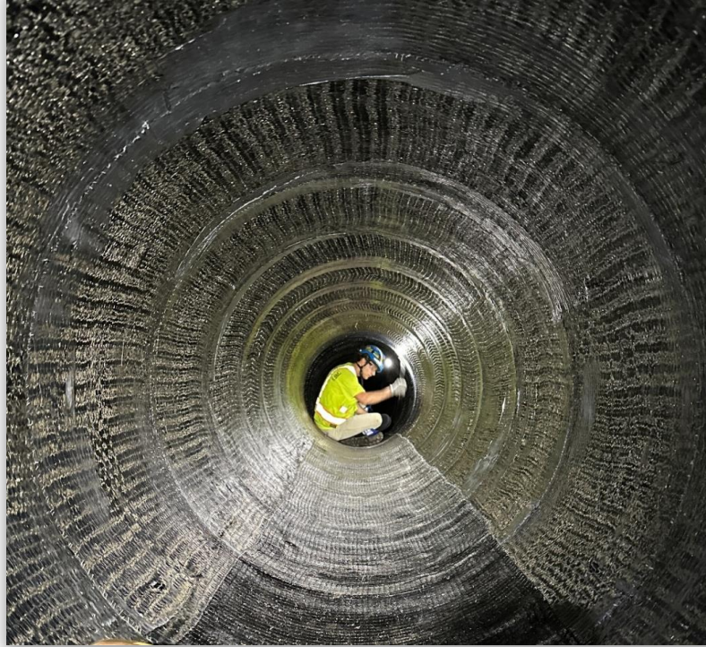
Testing for Voids
