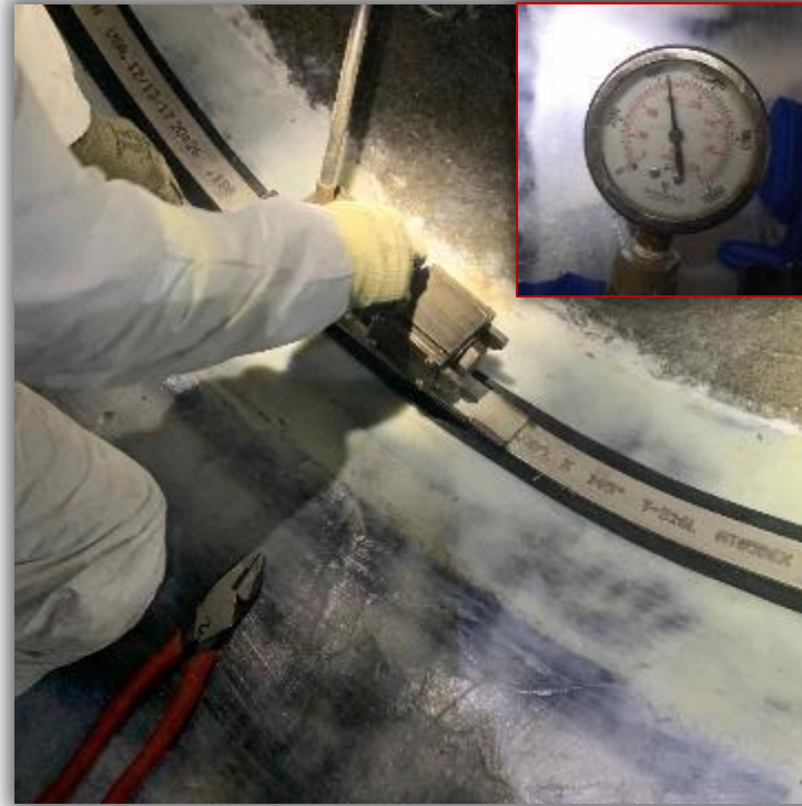
Compression Ring Installation at Terminations
