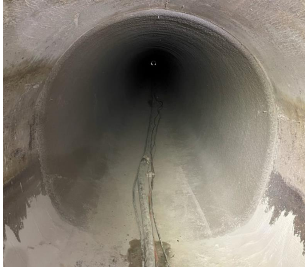
Geopolymer Application at Transition
