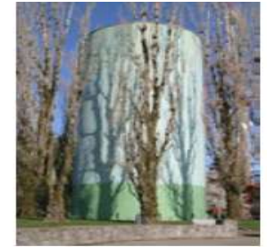
66 Tanks and Reservoirs
