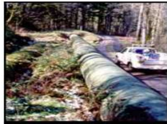
100+ miles of large pipe
