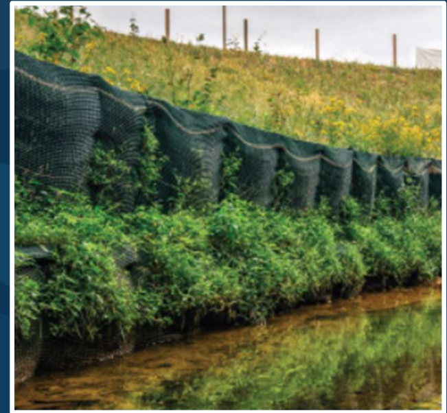
Soil Filled Gabions
