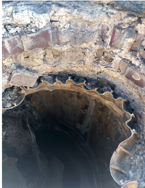
Water Infiltration, Delamination, Structural Integrity Lost
