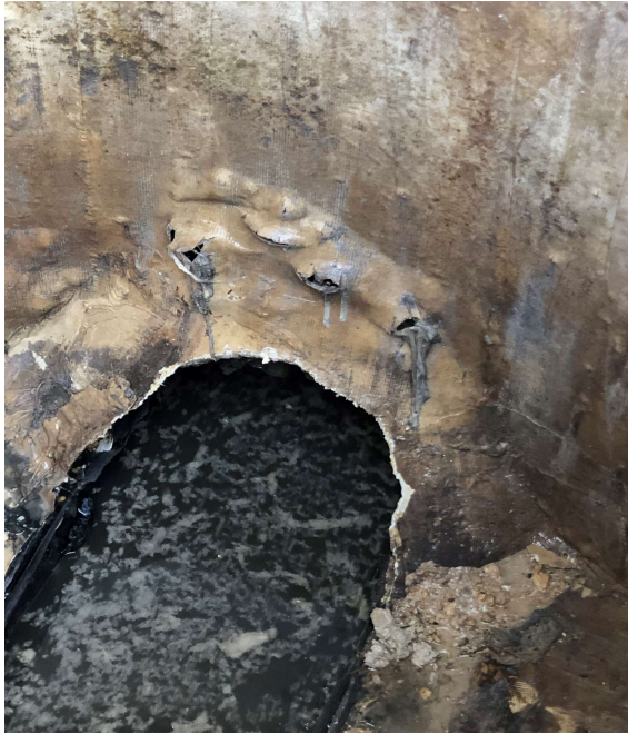
Water Infiltration, Delamination, Structural Integrity Lost
