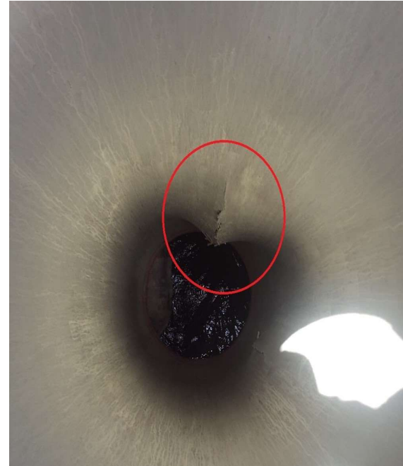
Water Infiltration, Delamination, Structural Integrity Lost
