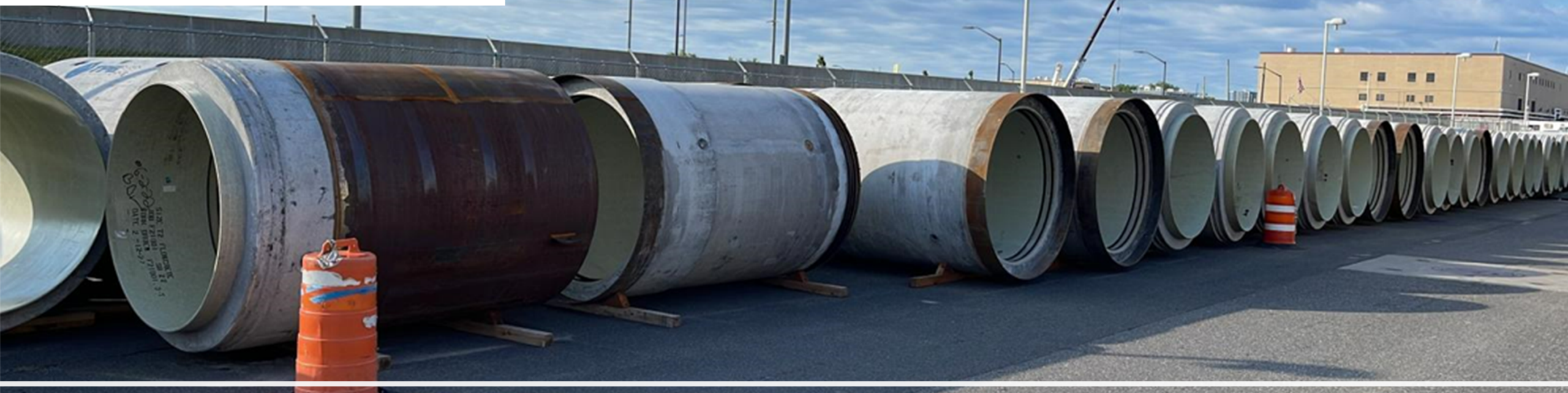
RCJP Considerations – Corrosion – Flowcrete
