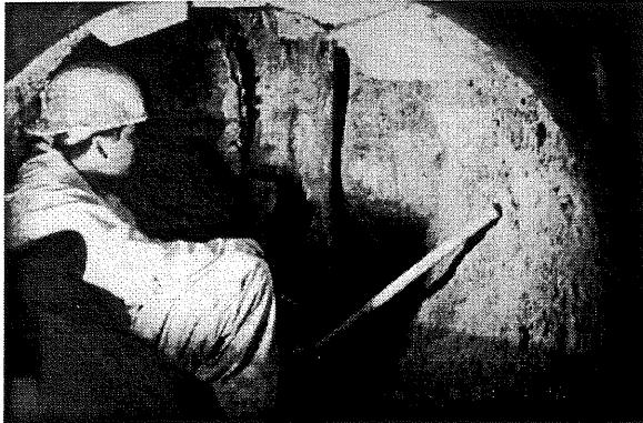
Well, Oh Well - Hitting Casing 40' Deep
