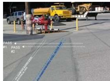
Figure 2a: A Job Site with 2 steel Pipelines
