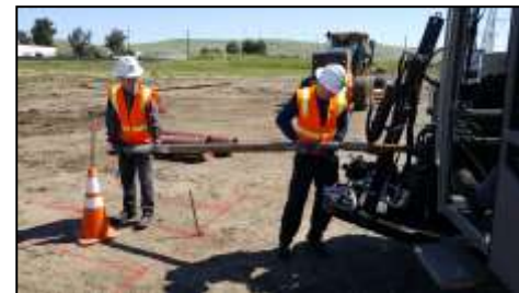
Figure 2: ORFEUS being installed on HDD rig.
