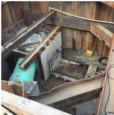
Figure 6: Reaction Wall on the Walnut Street Side (Photo by Kennedy/Jenks)
