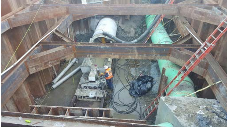
Figure 5: Sewer bypass in jacking pit (Photo by Kennedy/Jenks)
