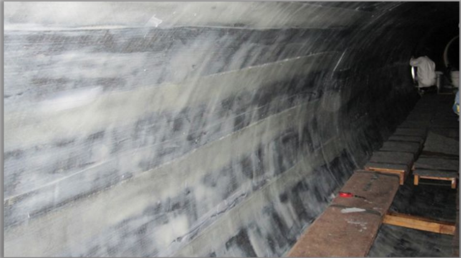
Installation of a watertightness layer
