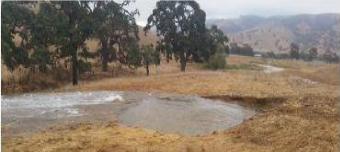
Site of ruptured pipe
