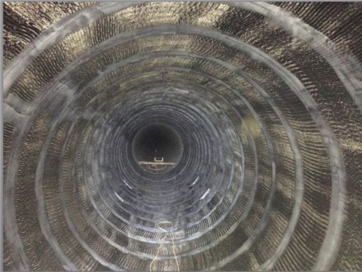
Completed CFRP lining
