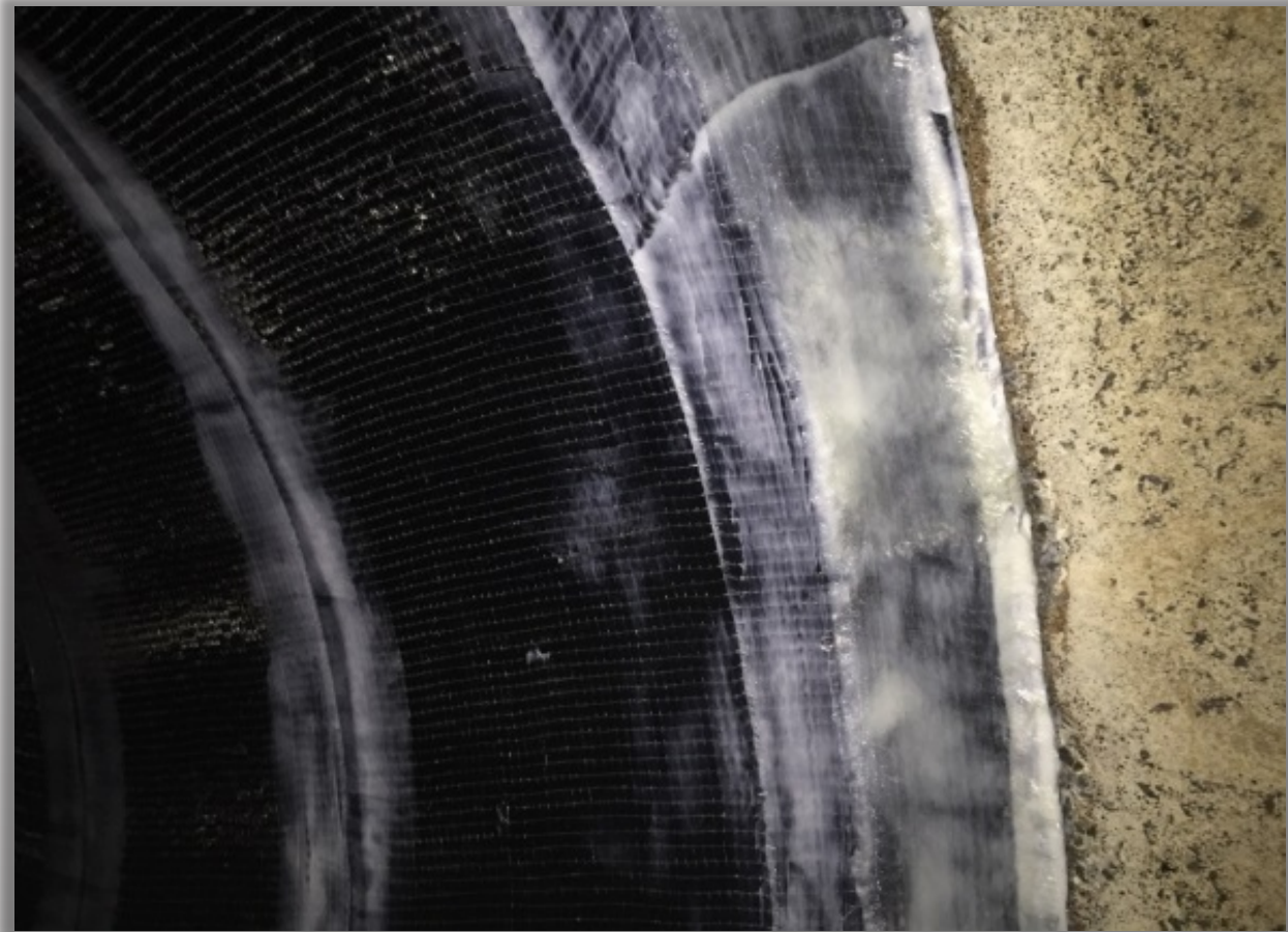
CFRP layers at end detail
