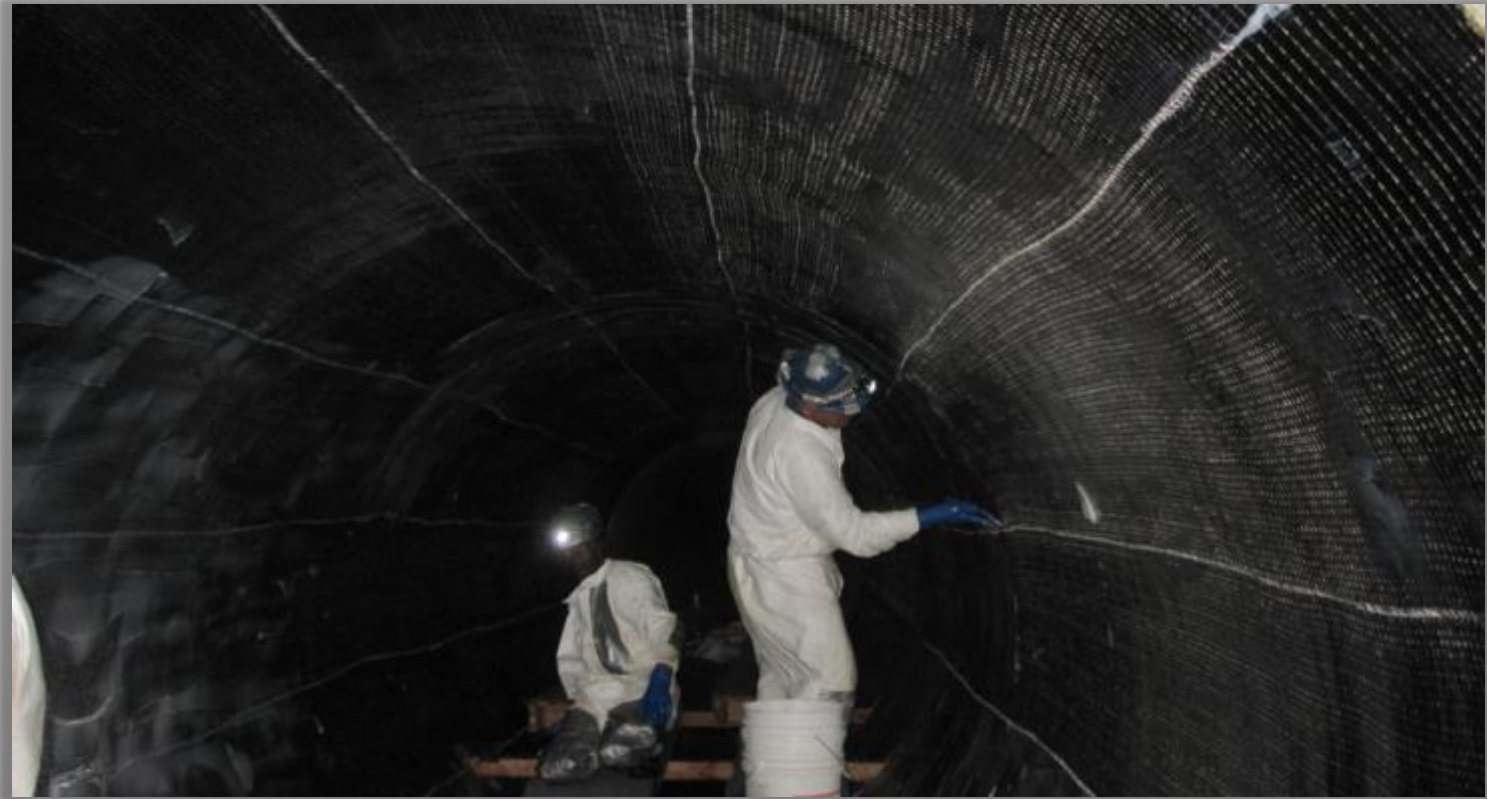
Installation of longitudinal layer of CFRP
