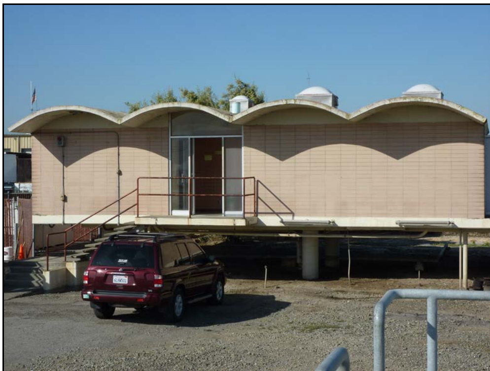
Figure 2 - The Spreckles Pump Station Administration Building was constructed on piers to protect the electrical equipment from flooding.
