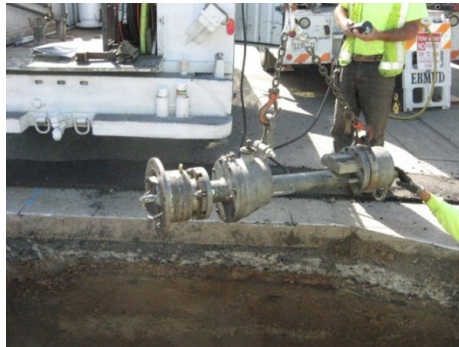
Figure 2.12 – Pipe Tap Machine
