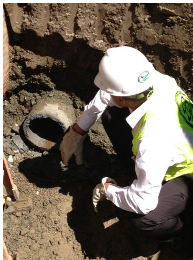
Figure 2.14 – AC Pipe Excavation
