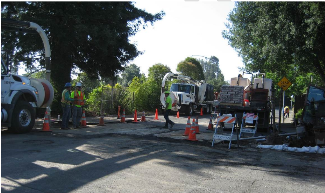
Figure 7. Maintaining access across a cul-de-sac while avoiding high pressure gas mains and significant trees for the F Street crossing.
