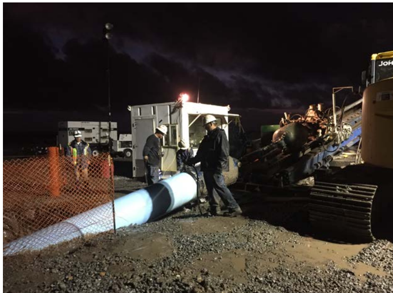
Figure 10: Completion of Pullback.
